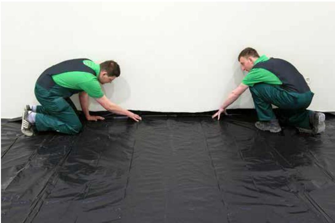
Floor installation should begin with the laying of the underlay with edges touching (but never overlapping). This does not apply to some floor planks which are laid with 2 mm expansion gaps between individual planks and a 10 mm expansion gap by the wall. Natural materials should be used as underlay, such as those offered by econfloor.
