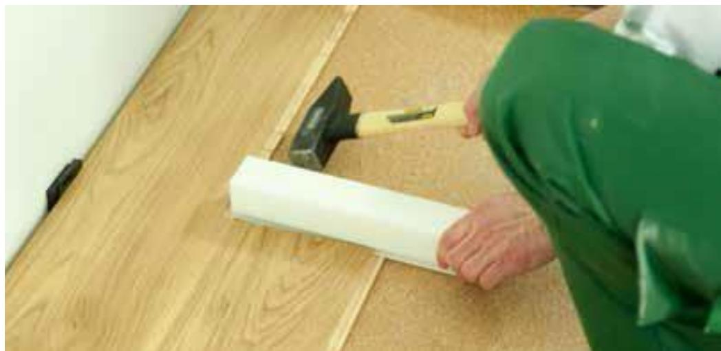
Cut the tongue off the first row of floorboards and place that side to the wall. Connect the individual floorboards on their shorter sides (ends) using the hammer and tapping block. Trim the last floorboard, remembering to keep an expansion gap from the wall.
